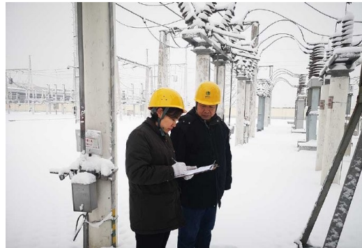
Figure 2. Traditional manual inspection
