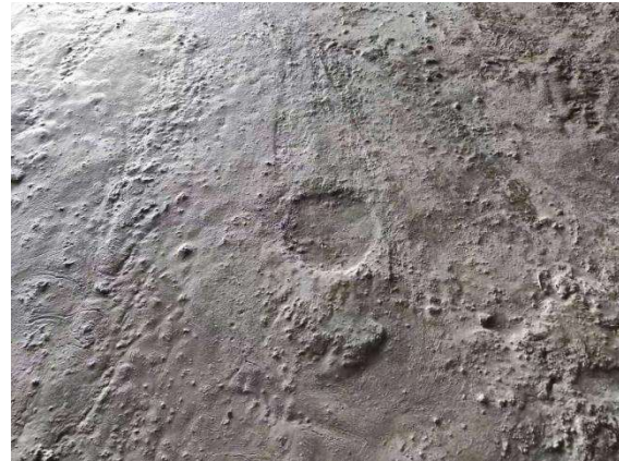
Figure.4 Grouting to complete
