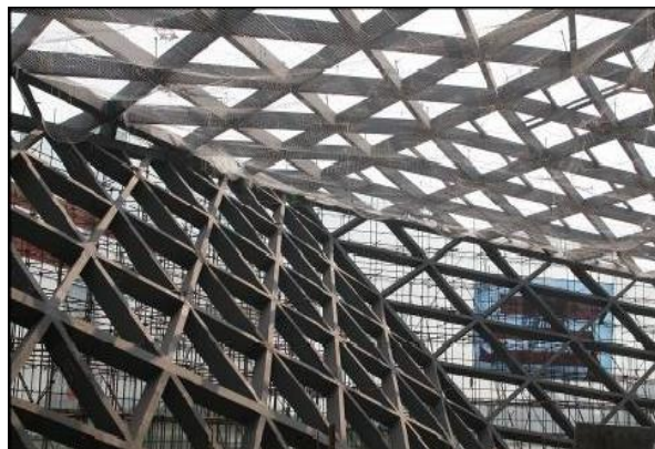
Fig 3. Concrete skeleton under construction (Zaha Hadid Architects,2009)
