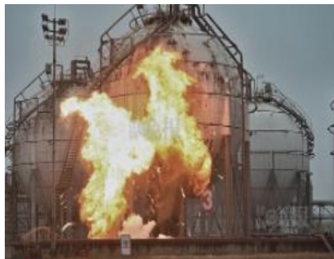
(b) Fire caused by hazardous gas leakage
