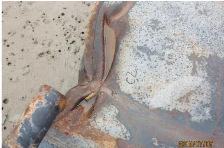
Figure 9. Site map of structural damage in the ship
