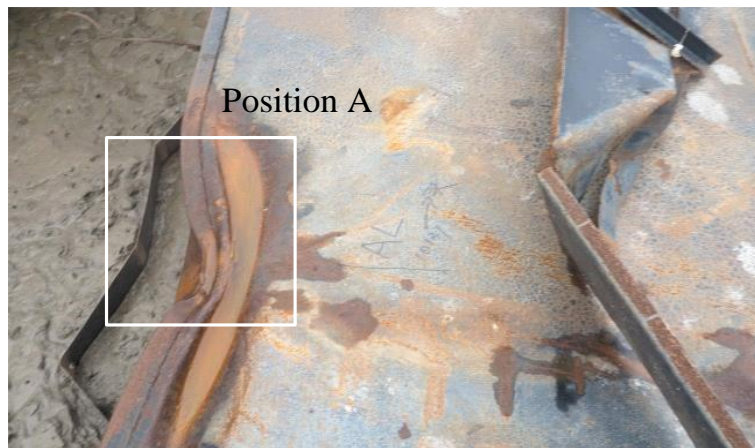
Figure 2. Position A structure destruction
