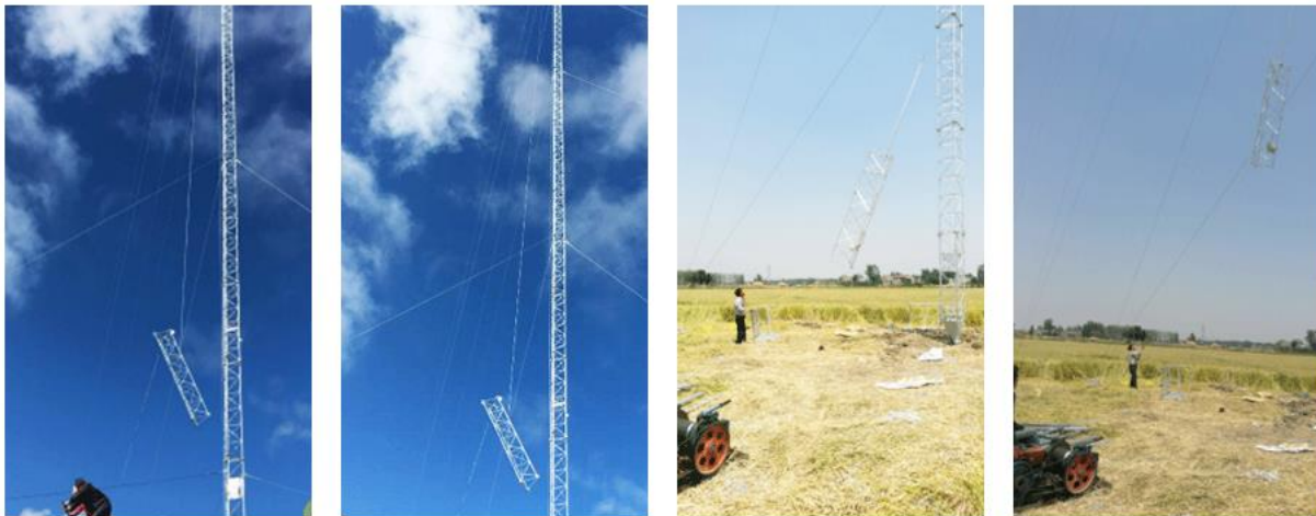
Figure 5. Schematic diagram of active descending tower construction
