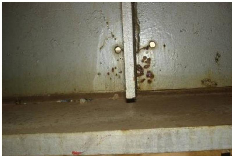
**Fig.1** The crack is caused in web space
