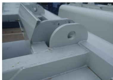
Figure 4. Lifting mechanism support position
