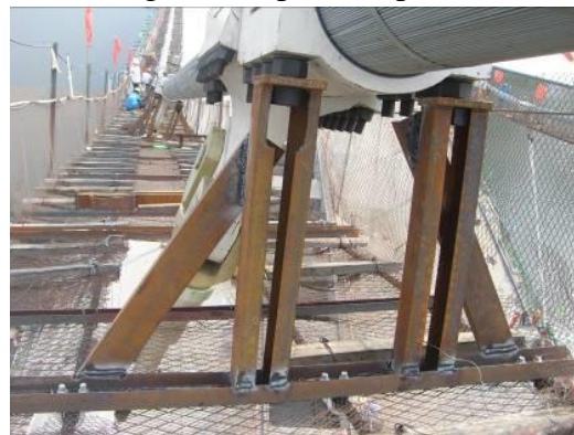
Fig. 6 alignment adjustment of catwalk
