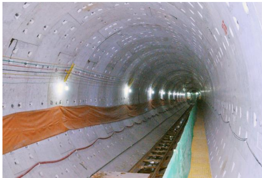
Fig 6. Chart of tunnel duct pieces Fig 7. Diagrammatic sketch of measuring points on segment ring To finish the measurement of duct piece posture, four joints on the left , right, top and bottom of segment ring are regarded as layout location of mark points, as is shown in Fig 7. On the tunnel duct pieces, set a group of measuring points per 5 rings. Measuring points are painted on reflecting marks, which is fixed on expansion bolt. Later, someone installs them on the tunnel duct pieces.
