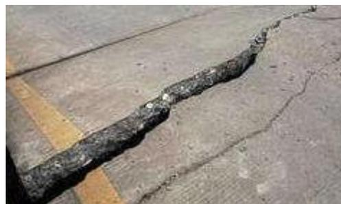
Fig.4 slab rupture
