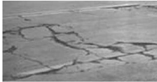
Fig.2 Reticulate crack
