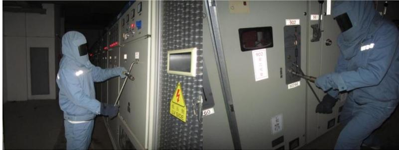
Fig. 4 The actual operation figure using the developed multifunctional insulated operating rod
