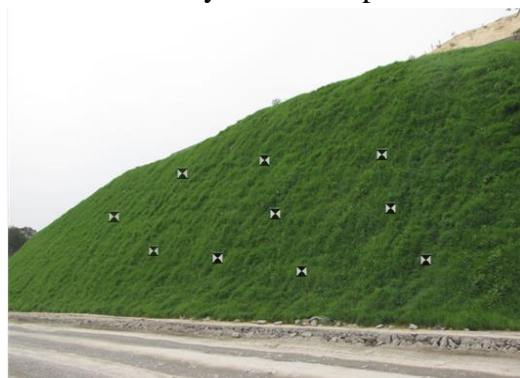
Fig. 2 Monitoring of highway side slope body
