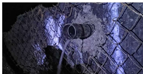
Figure 7. Physical photo of K2 inspection hole effluent
