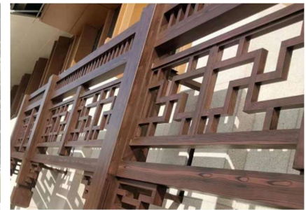
Figure 2. The Wood Grain Paint Used in the Railings of the Ancient City of Xi'An
